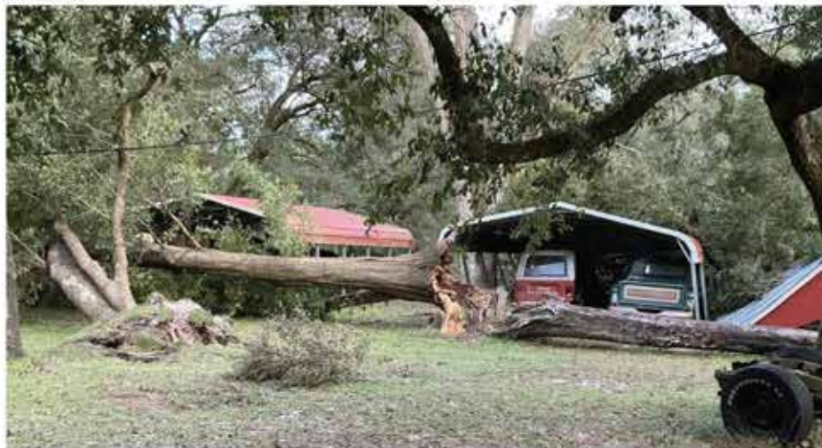
SWCE's line crew captured a photo of the damage in Florida following Hurricane Milton.
