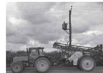
Farm operators are encouraged to look up and look out for power lines as they spray their fields. Steele-Waseca's wholesale energy provider, Great River Energy, has already recorded two incidents this year.
