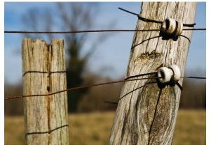
Electric fences are specially insulated from the ground and can pick up an induced charge from transmission lines. the charger unit is connected to the fence; however, when the charger is disconnected either for maintenance or when the fence is being built, a small shock may be produced. Contact your local electric cooperative for assistance. Typically such a shock can be prevented by:
