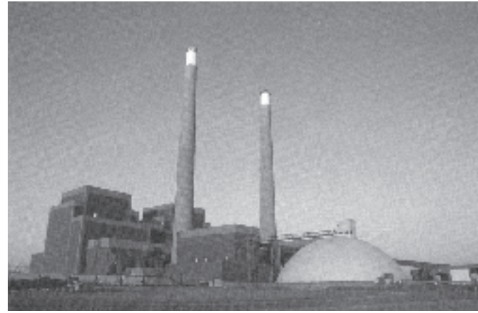
Fly ash collected at Coal Creek Station near Underwood, North Dakota, is stored in a dome (pictured at right) before it is sold for beneficial use. (Photo courtesy of Great River Energy)
