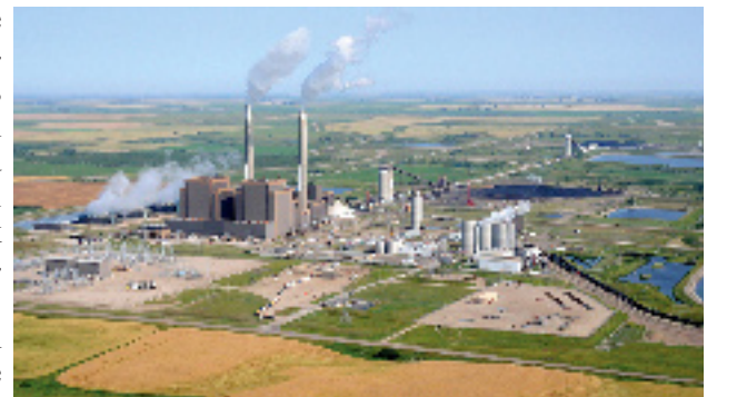
An aerial view of Coal Creek Station near Underwood, N.D. (Photo courtesy of Great River Energy)
